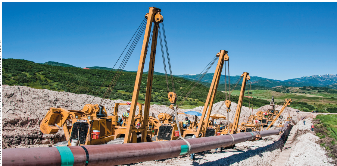
PHOTO COURTESY PIPELINE MACHINERY INTERNATIONAL
